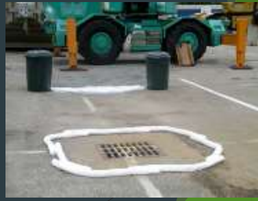
▶ Absorbent Booms Around Drop Inlet
